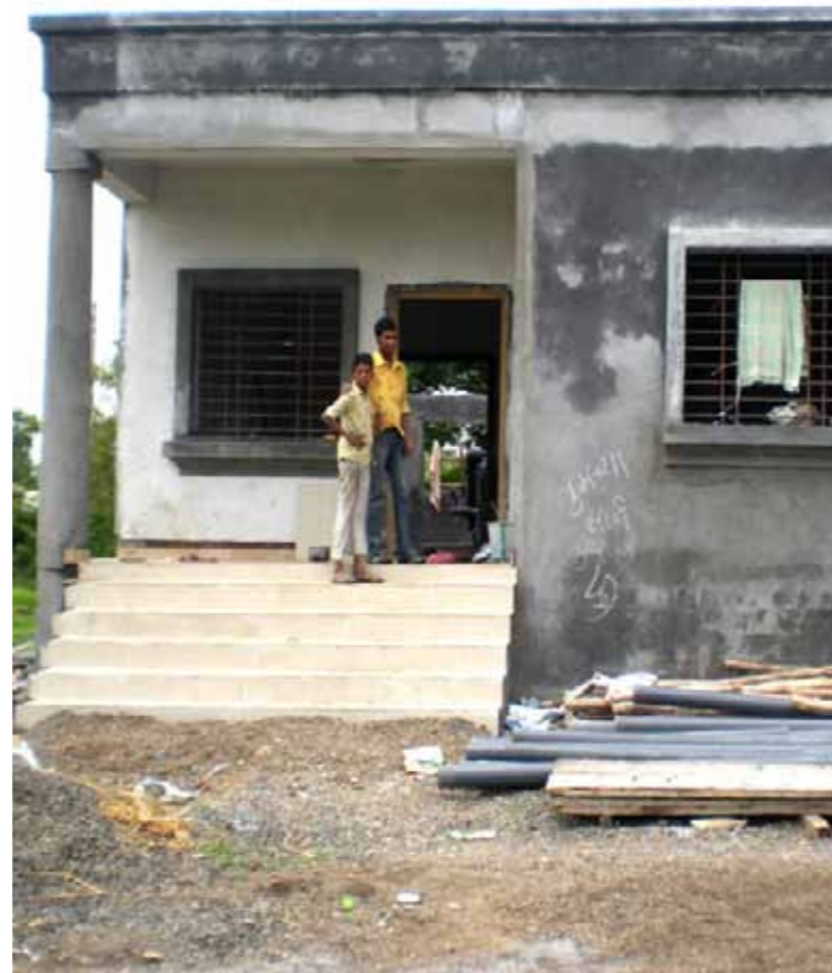
Quarters for Nurses- Construction in Progress
