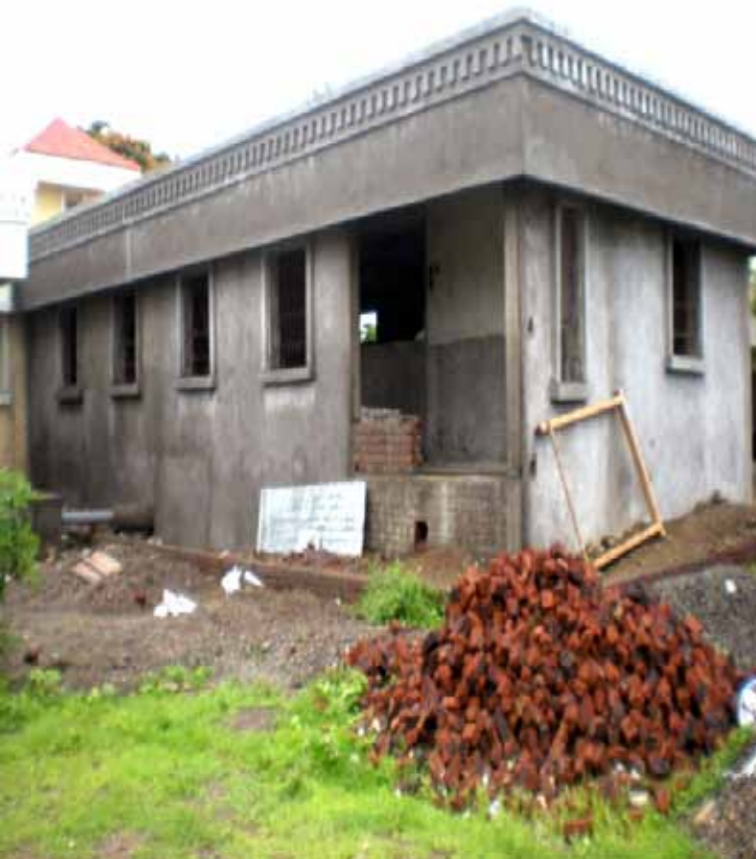
Post Natal Care ward - Construction in progress
